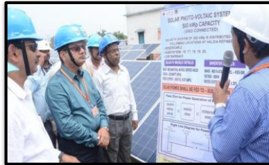
Rooftop Solar Project IOCL (Haldia & Panipat Refinery)
