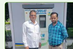
Gym Khanna Service Station BPCL Delhi
