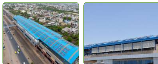
Solarized Maujpur-Babarpur Metro Station with a 1 MW setup on the tin shed.
