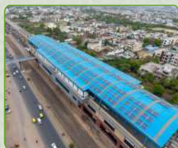
Solarized Maujpur-Babarpur Metro Station with a 1 MW setup on the tin shed.
