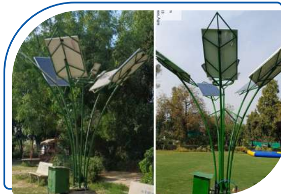
Glimpse of UPNEDA Solar Tree Project
