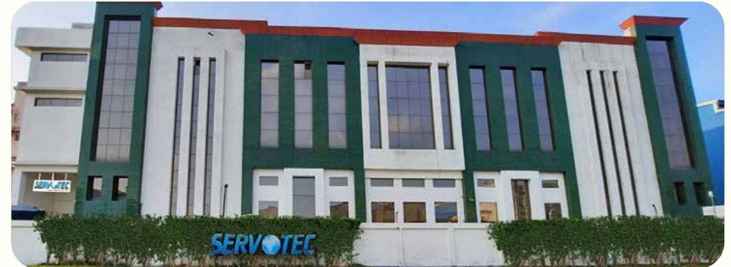
Lithium-Ion Battery Assembly & Testing (Home ESS, E-Rickshaw, BESS)
